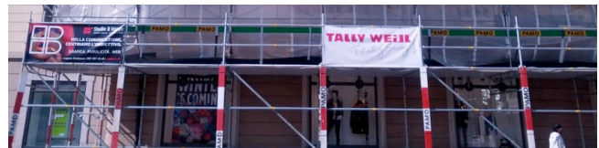
Figure 4 - An example of scaffolded poster arrangement on construction frame (PCF)
